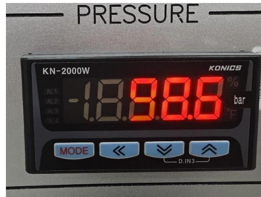
Figure 17) Photo of test condition (Water pressure)
