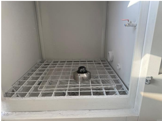
Figure 5) Photo of the specimen installation
