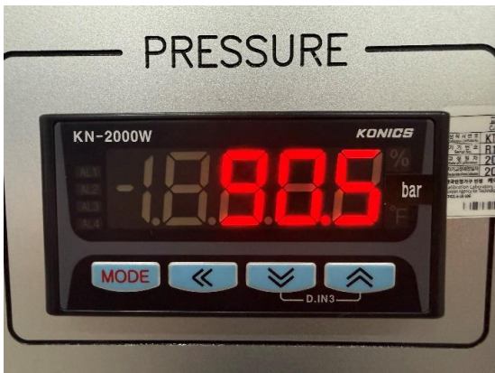
Figure 17) Photo of test condition (Water pressure)
