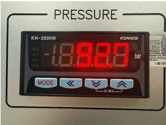
Figure 17) Photo of test condition (Water pressure)
