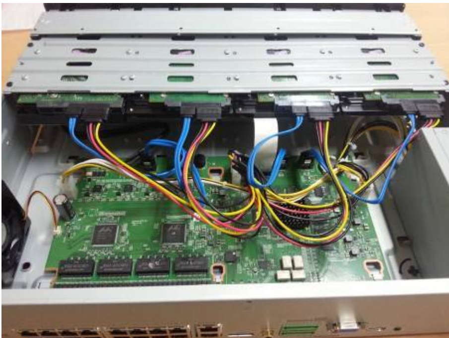
<Photo 8 > Inside view 1
